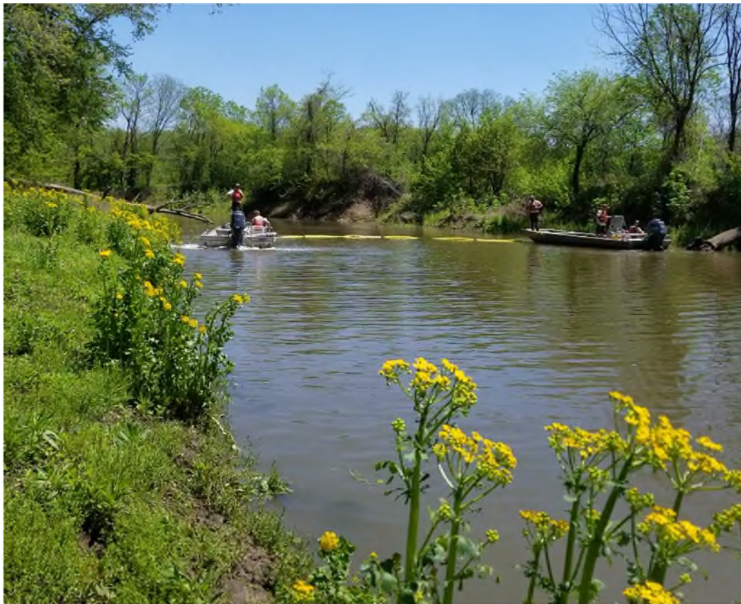
Figure 2. Flexible “Scare Curtain” being towed between two boats. White weighted 7inch strips of sun-shade fabric extend from the floats to the bottom of the tributary.
